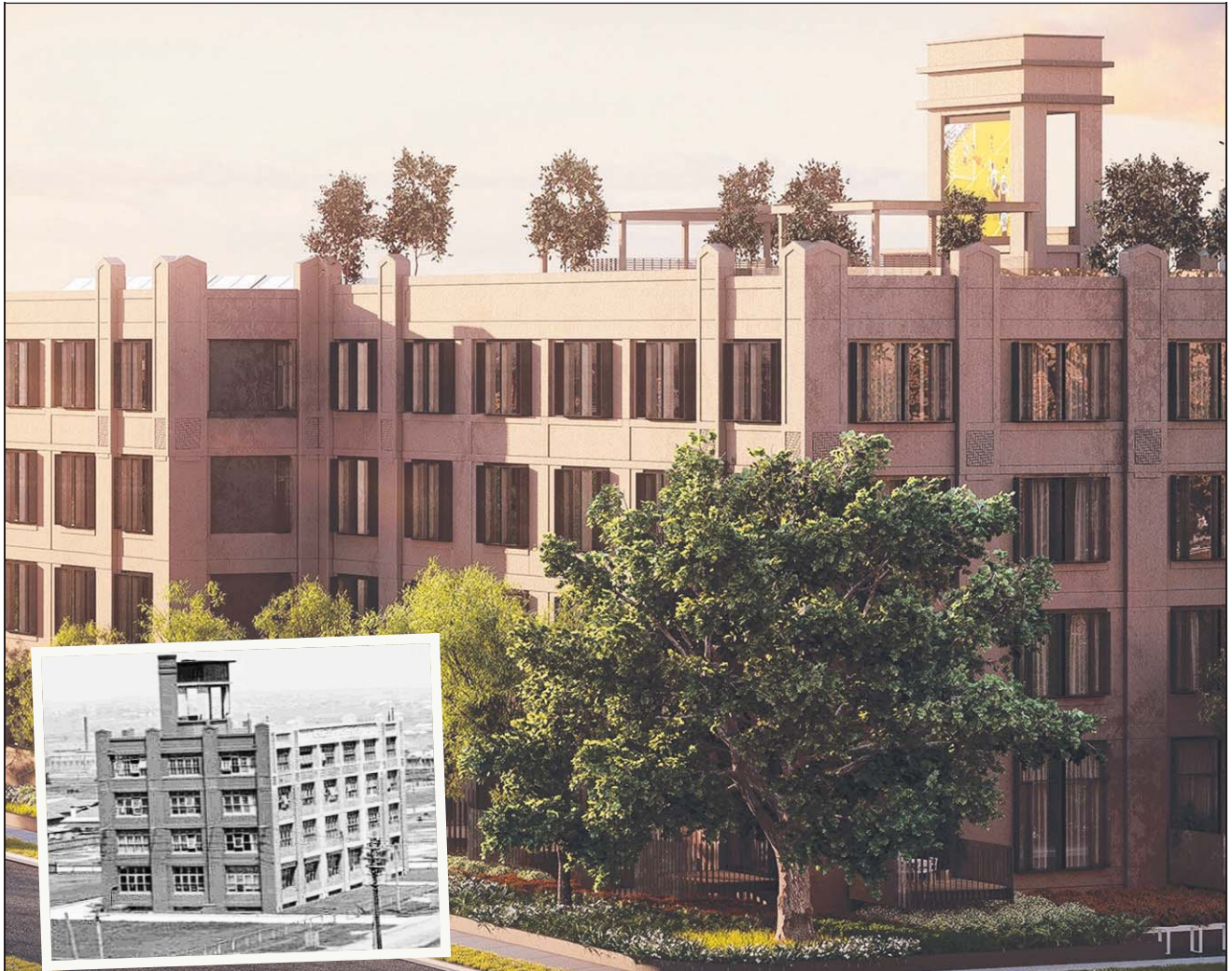
The Wrigley's Factory (inset in the 1920s) reimaged as modern apartments with a rooftop cinema.
