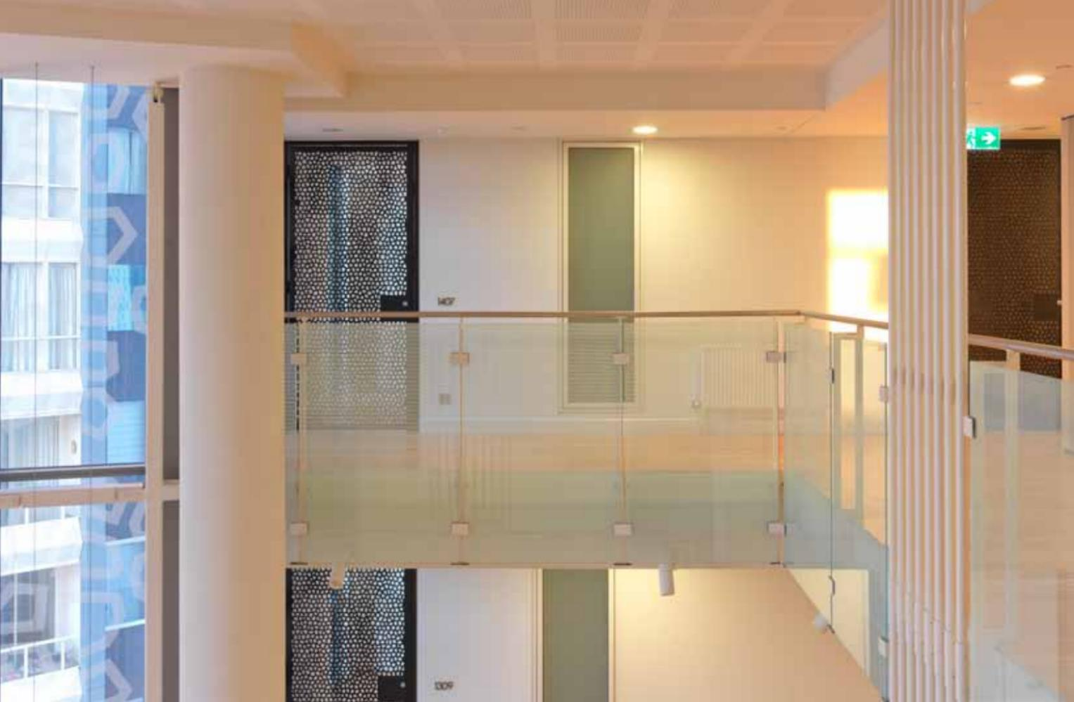
**Top left** To improve the cross ventilation, each apartment has an exterior lobby behind a lockable gate with an aerated metal screen.
